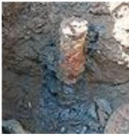
The corroded plate (left) is of copper. This shows that the common belief that copper electrodes will not corrode is not true.
